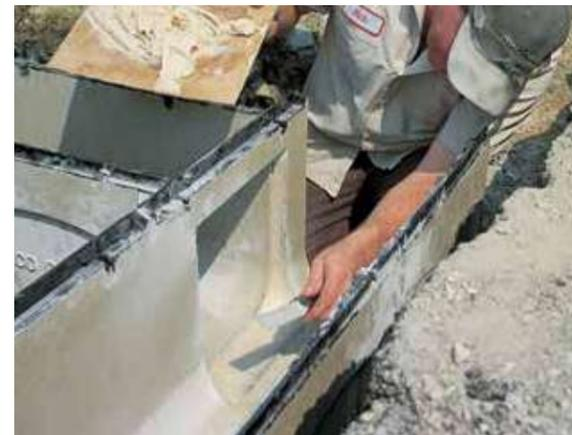
ACO channels are supplied with a Sealant Groove as standard. This provides a groove that can be filled with an appropriate flexible sealant to create a watertight joint. This is particularly important with elevated slabs and where liquids may contain chemicals or oils.
